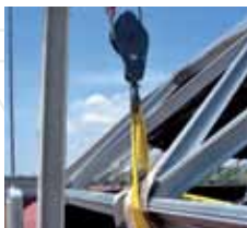
Lifting with grip hoists
